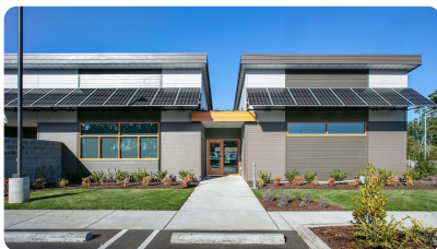
Florence Public Works Public Works Architecture Oregon —Sco
